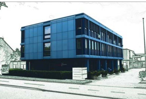
Administration and production facilities, Headquarters Winterthur / Switzerland
