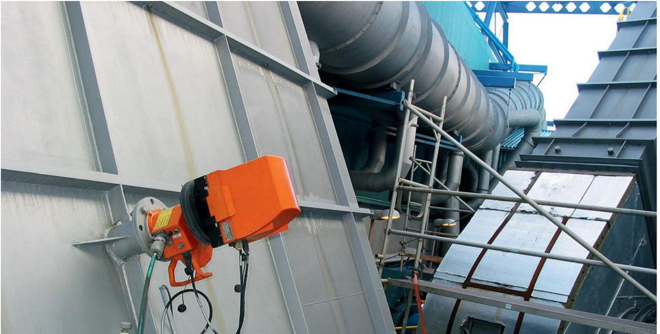
Measuring difficult, selective gas components such as ammonia ( $\text{NH}_3$ ), hydrogen fluoride (HF), and hydrogen chloride (HCl) is a major challenge for process analysis and emission monitoring. The GM700 in-situ gas analyzer opens up new options here. With unparalleled flexibility – without the need for test gases.
