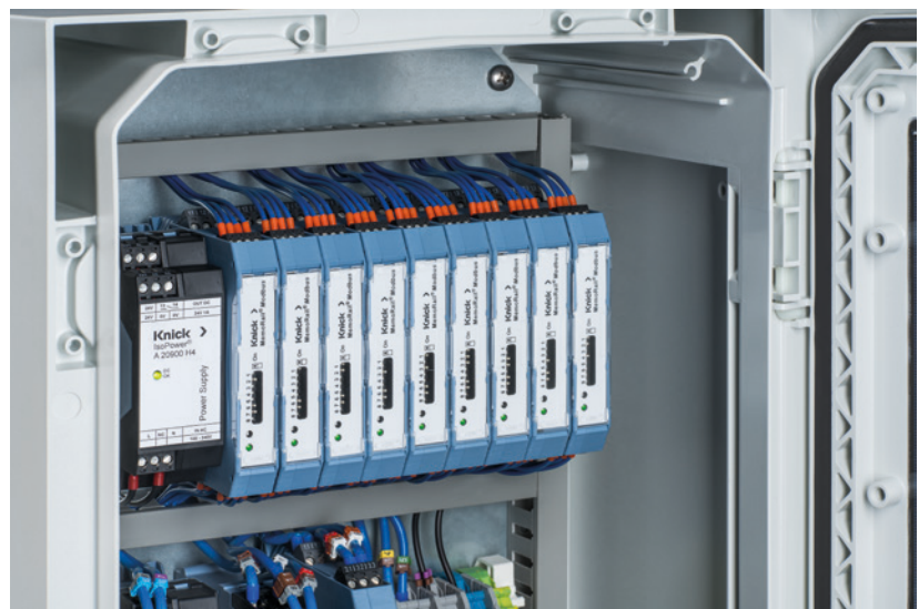
Installation in a control cabinet
